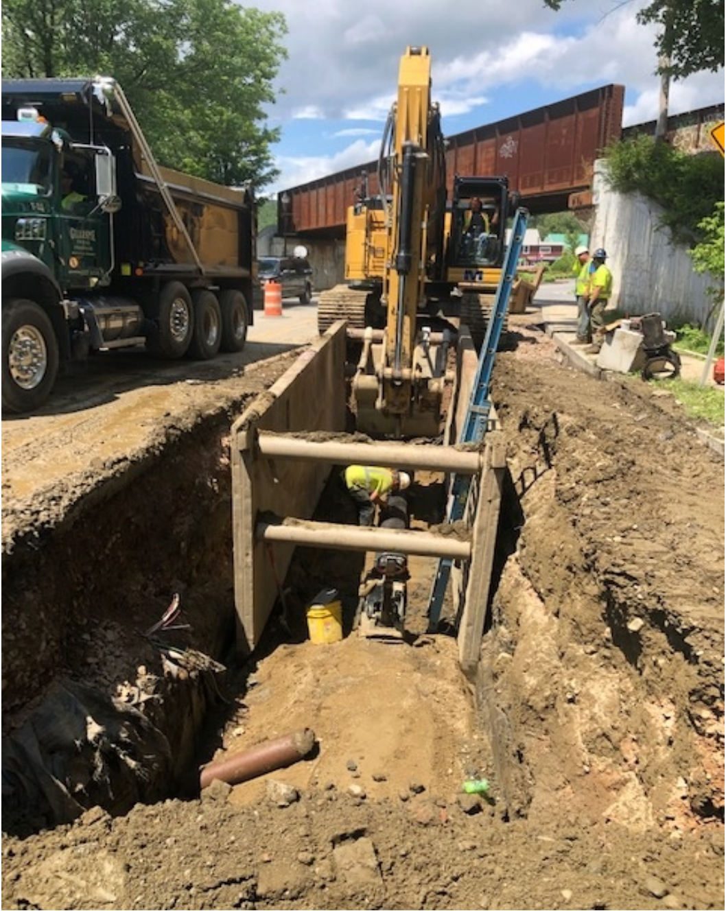
Alternating one-way traffic used for deep utility installation.
