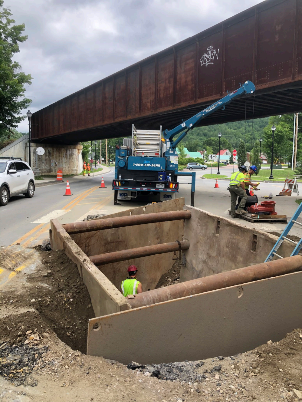
Alternating one-way traffic used for deep utility installation.
